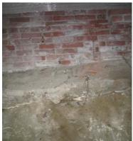
Water was observed in certain areas of the Basement floor (Photo). The perimeter brick foundation walls also show signs of moisture absorption (efflorescence present). Moisture related damage is evident at the base of a number of brick masonry support piers; repair is recommended. Basement/foundation drainage issues should be evaluated by a Geotechnical Engineer, in conjunction with the above recommended stability review.
