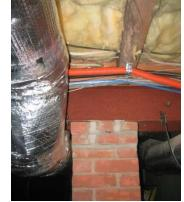
Foundation walls are brick masonry construction, with a stone (gneiss) facing above grade. Perimeter foundation drainage does not likely exist. .
