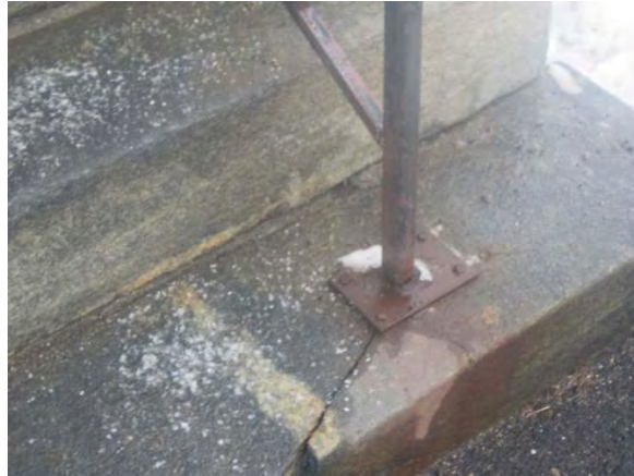
Figure 1. Several stair treads have been destroyed by rusted railing mounts that were not maintained and caused the stone to crack. Each stairway has heaved, treads have cracked and failed because moisture was allowed in and, over decades, the brick masonry support structure beneath deteriorated and failed.
