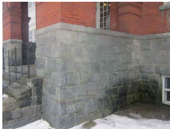
Figure 2. Algae and other biological growth is evidence of roof and site drainage issues, particularly on the northern side of the building. The introduction of gutters will alleviate this issue. The growth can be safely cleaned with any number of commercially-available, anti-microbial solutions.
