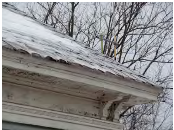
Figure 4- West Elevation of Ell showing poor roof edge detail.
