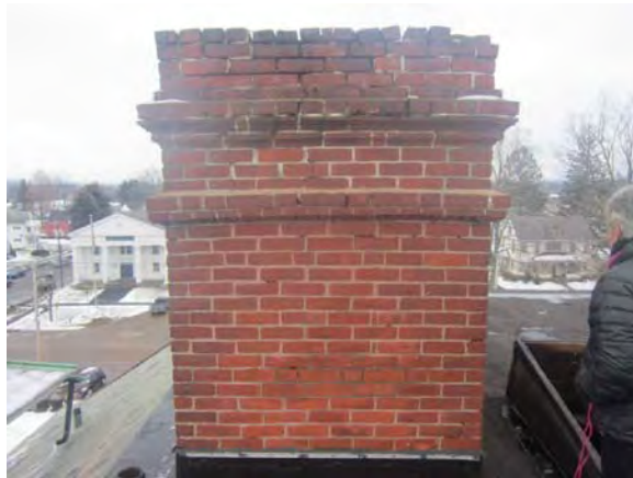
Figure 19. The chimney stack has not been maintained. A section of the sheet metal cap is missing and has allowed the top three courses of brick to fall into disrepair. These courses must be re-laid and sections of the stack repointed with an appropriate mortar.
