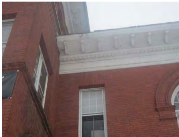
Figure 11. Broken slate at the eaves allowed water runoff to damage the cornice. The damage to the slate may have initially been caused by icy snow sliding off the tower roof, above.
