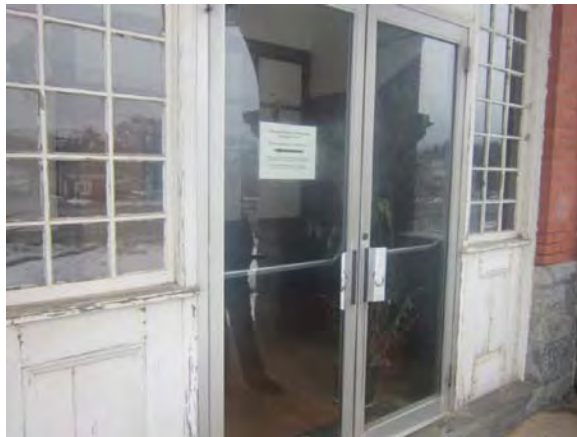
Figure 20. The aluminum entry doors on the west porch are functional. Windows, panels and trim are in need of restoration.
