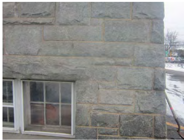
Figure 8. Extensive cracking is visible through the mortar joints at the southeast corner of the building (typ.) The installation and monitoring of tell-tales will help determine if movement is occurring or not. Cellar window. ($15b) is missing storm inserts. Two panes of glass are broken and “boarded closed.” The missing storms are allowing precipitation to rot the sill and window.
