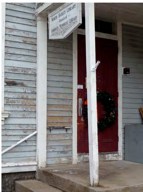
Figure 14- South Porch Elevation showing dislodged and deteriorated post.
