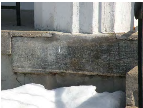
Figure 2- West Portico showing separation of stone and concrete.
