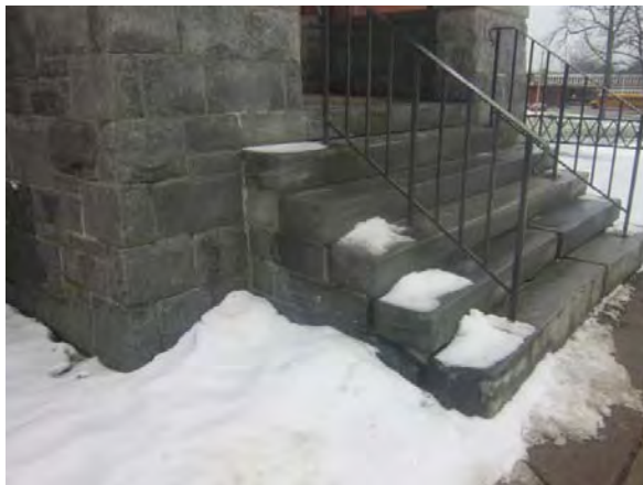
Figure 5. The stairs of the northern porch have failed. Beneath the steps are stringers, typically made of brick. When the joints between the treads are not kept pointed or closed with appropriate adhesive mastic, water gets inside. The bricks supports are destroyed and, over the years, the less-supported treads sag. The stone steps crack and become askew.
