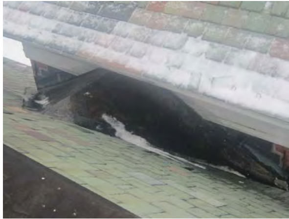
Figure 16. The cricket behind the tower. Like the sidewall detail discussed in photo two, above, inappropriate materials and methods have been employed in an effort to prevent water infiltration. Slate roofs will last for hundreds of years. Replacement of sheet metal flashing assemblies, like this, after one hundred years of service life are considered part of the maintenance of a slate roof system.
