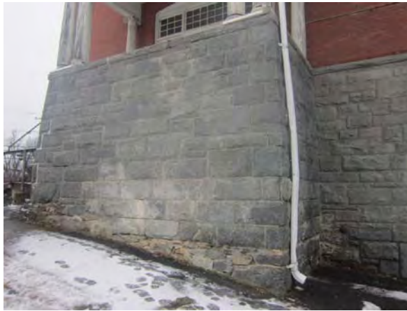
Figure 7. Water infiltration, detailed in the preceding photo, has compromised the mortar joints on this side of the porch. Without proper attention, in short time this side will start to bulge out and rebuilding will be necessary. Note the exposed portions of the once sub-grade rubble foundation wall. Erosion and/or settlement has presumably lowered grade since the date of original construction.
