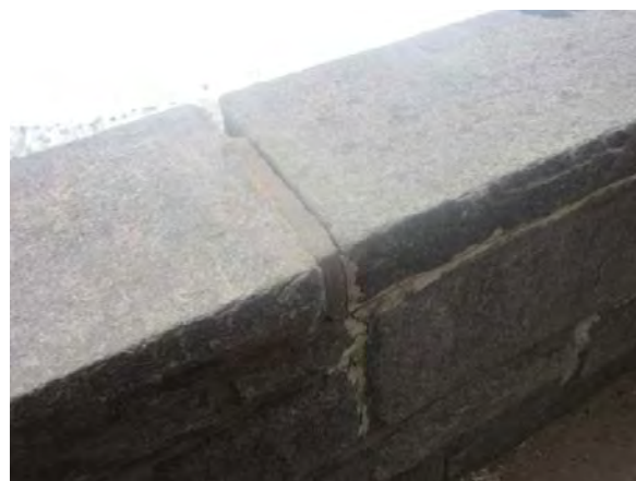
Figure 6. A failure to keep cap stones pointed or closed off with appropriate adhesive mastic will allow water inside. That water, during freeze-thaw cycles, will destroy mortar joints and, ultimately, the structural integrity of the wall will be compromised.
