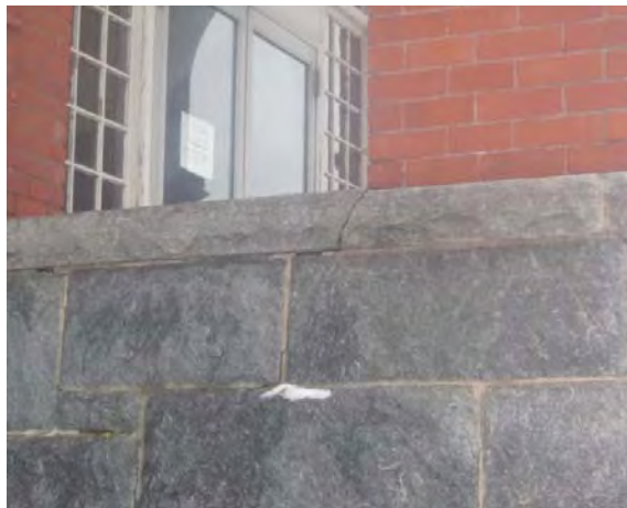
Figure 23. The cause of the crack in this cap stone, on the northern porch, is not immediately evident. There are no signs of failure elsewhere in the tower, and one corner is supported above this section of the porch. The use of tell-tales will indicate if any movement is taking place. It is most likely that some minor settlement occurred during or soon after construction. The result caused the crack in the cap to appear thereafter.
