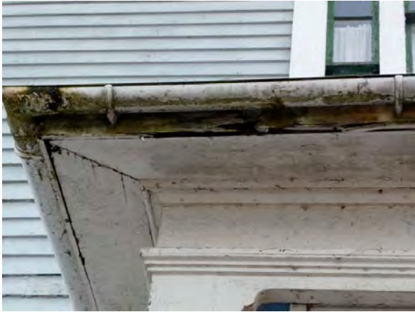
Figure 8- West Porch roof deterioration at eave and cornice.
