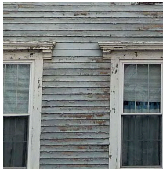
Figure 13- South Elevation showing bow in exterior clapboards.
