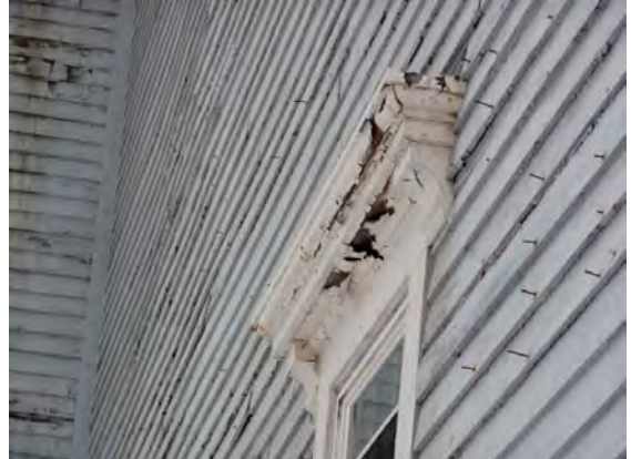
Figure 3- East Elevation showing just jacking at clapboard nails.
