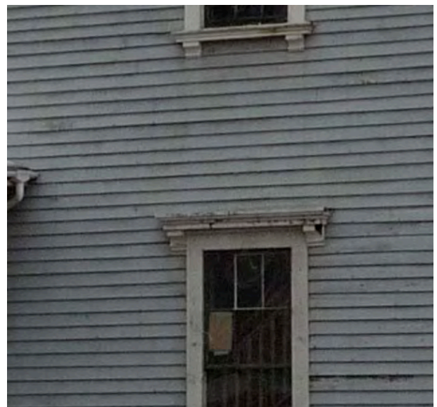
Figure 11- West Elevation window bracket requiring Dutchman repair.
