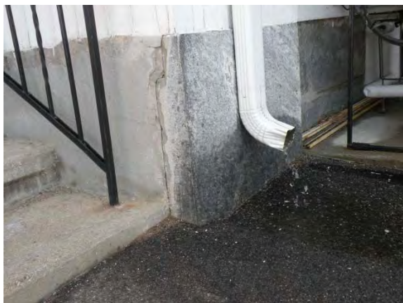
Figure 1- Southwest corner showing stone joint.
