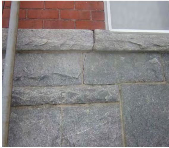
Figure 22. A failure to maintain the mortar joints of the belt course allowed precipitation to infiltrate on the northern elevation and exacerbating movement. Note crack in the stone of the foundation.
