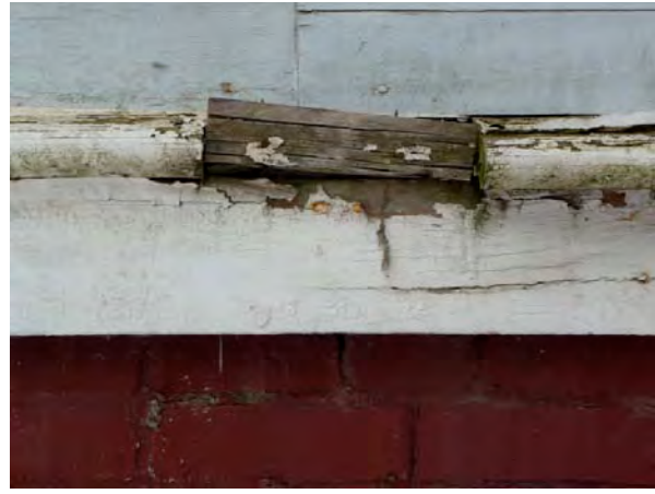
Figure 19- North Elevation showing deterioration at water table from roof run-off.
