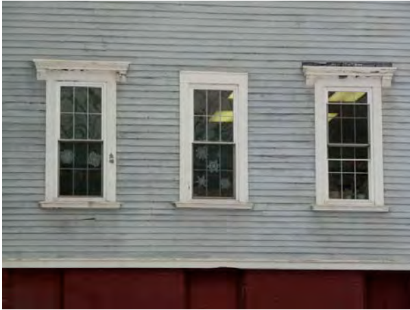
Figure 17- East Elevation showing missing window hood.
