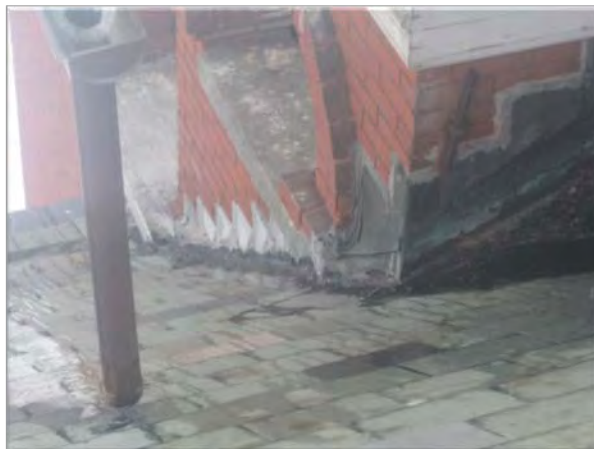
Figure 15. This picture details the stop gap measures that have been employed at the masonry sidewall and cricket. The roofing tar contains bituminous by products that actually accelerates the deterioration of the copper sheet metal. The repairs are inappropriate, unsightly, and destroying adjoining slate.
