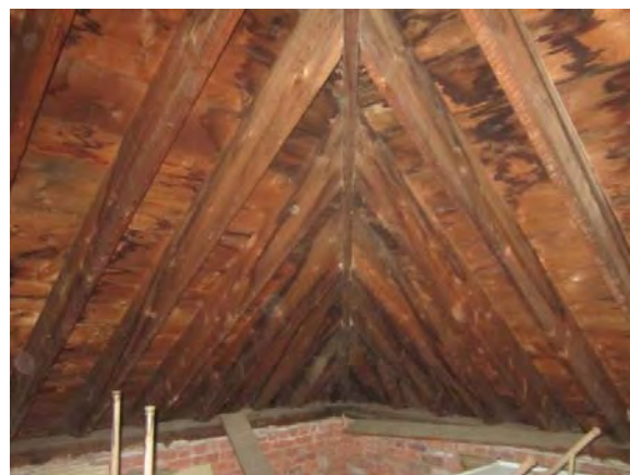
Figure18. Roof structure. The structural members of the roof frame are in very good condition. No deflection or rotting was detected. Water staining, as shown in this image, was most likely incident specific or related to a missing slate which has since been replaced.
