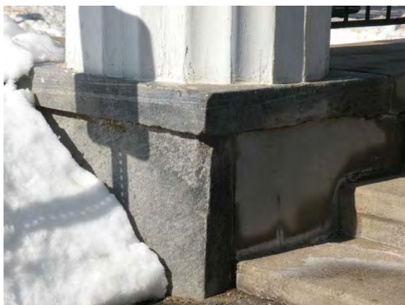
Figure 3- West Portico deteriorated parge coat.
