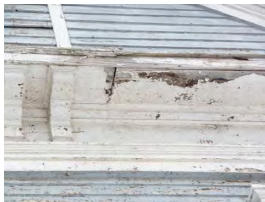
Figure 15- South Elevation at Ell showing deteriorated cornice and soffit at pediment.
