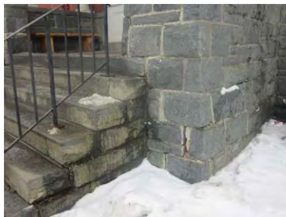
Figure 3. The stairs and abutting walls of the eastern porch. Failure to maintain mortar joints, particularly with cap stones, has allowed moisture to infiltrate. The infill freezes, expands, and forces facing stones to bulge outward.
