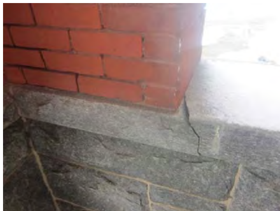
Figure 24. The porch side view of the crack discussed in Figure 23, above. Note the general deterioration of the brick mortar joints. Masonry will last for centuries if properly maintained. The repointing of mortar joints is critical to the longevity of a masonry structure.
