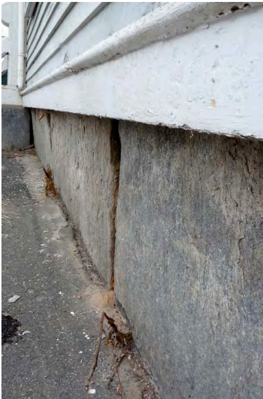
Figure 2- West Elevation showing minor shift of capstone, washed-out mortar and brick dust.
