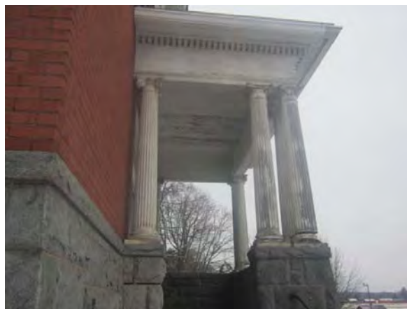
Figure 12. While the western porch requires the most carpentry-related work, its masonry is in better overall condition than the other two. The volutes of the capitals are missing or in poor condition some are askew from their plinths. One column is completely missing.
