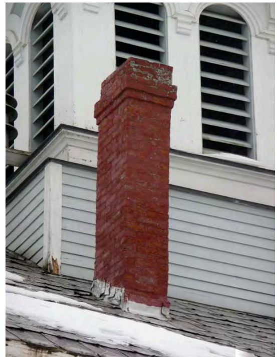
Figure 5- North Elevation showing roof flashing at chimney.
