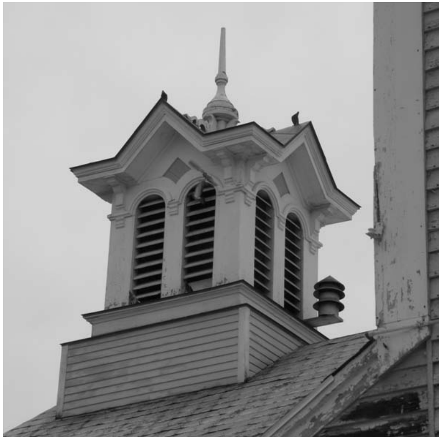
Figure 7- South Elevation of Cupola showing water damage from roof run-off.
