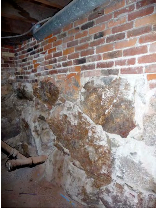
Figure 1- North Elevation at basement showing brick spalling.
