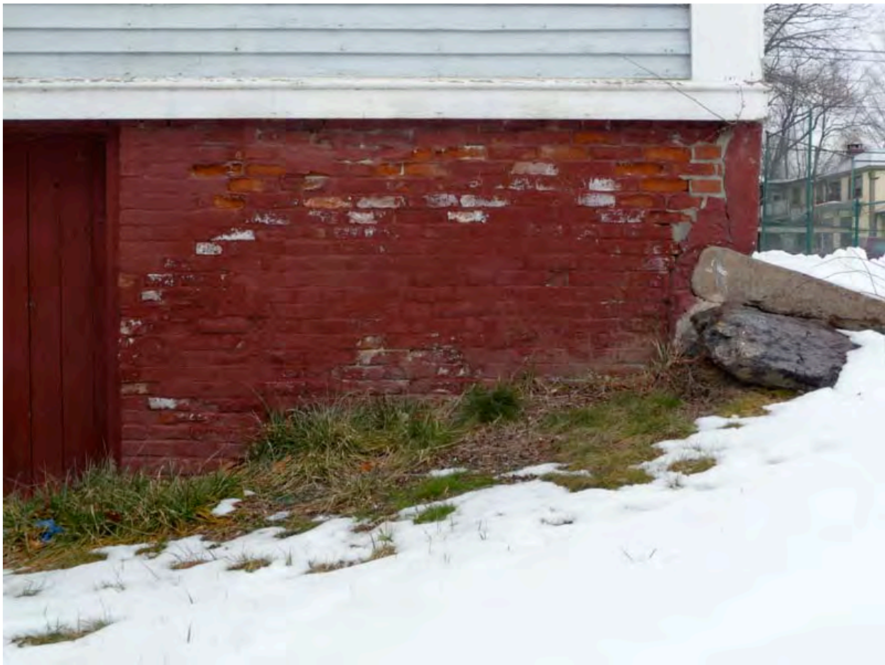
Figure 18- East Elevation at Northeast corner showing spalled brick, efflorescence and inappropriate repair at capstone.
