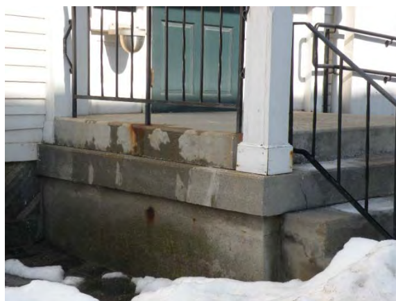
Figure 5- Crack at South Porch column.
