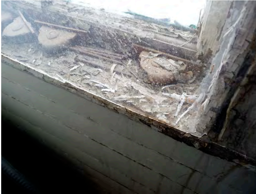
Figure 6- Interior window damage from condensation due to interior storm window.
