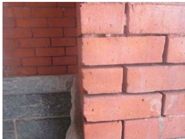
Figure 9. Detail of the deterioration of the mortar joints on the north porch. Some minor pitting of the face of the brick is detected, but not enough to warrant replacement of the masonry units. Again, the repointing of masonry facades is a maintenance-level action that will promote the longevity of the wall system.
