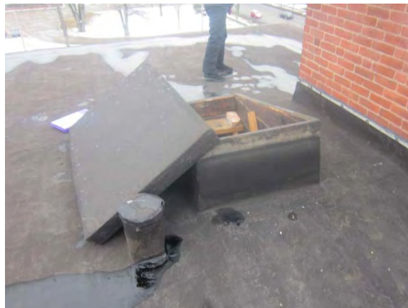
Figure 17. The roof hatch, curbing, protrusions, and condition of the modified bitumen roof all appear to be in good condition. These elements should be inspected quarterly for leakage and potential failures from the roof and the attic, underneath.
