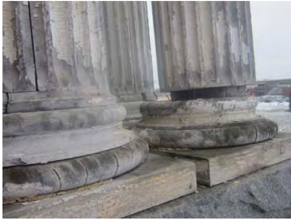
Figure 13. Detail of the column bases. Decades of neglect have allowed the columns to deteriorate to this condition. The fact that they have survived, even in this condition, is a testament to the quality of materials. Note the “alligatoring” (crazed and cracking) of paint in the flutes, an indicator of lead-based paint.
