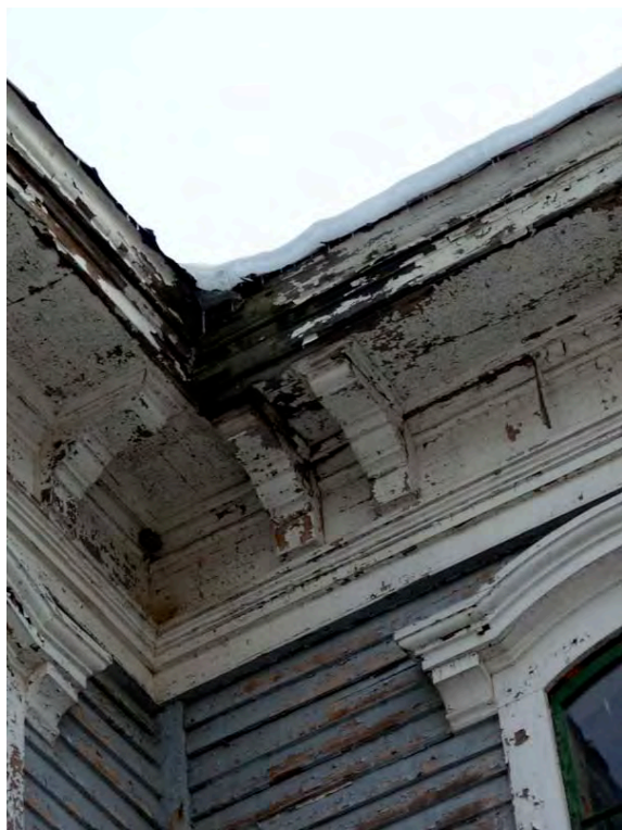
Figure 12- Cornice and soffit deterioration from roof run-off at the Southwest corner elbow.
