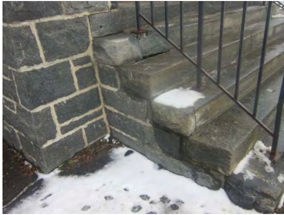
Figure 4. Sections of the eastern porch have been repointed with an inappropriate material by an unskilled person or persons. Improper installation and later maintenance of the railing system has allowed the wrought iron to rust and expand. This has caused wholesale destruction of the stair treads.
